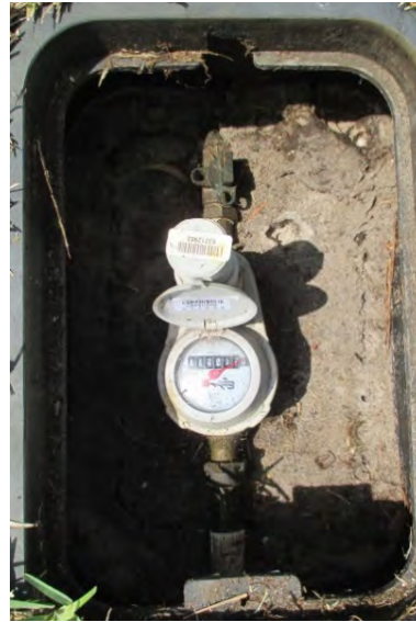
Water Meter inside a meter box
